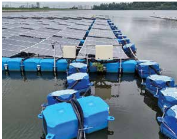
FIGURE 9.6 Vegetation growth due to the spreading of seeds by air, water, or bird droppings
