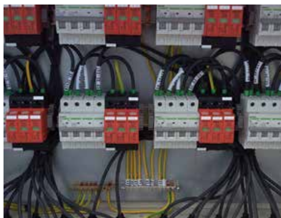
FIGURE 8.2 DC cabinet with surge protection devices (red-orange)
