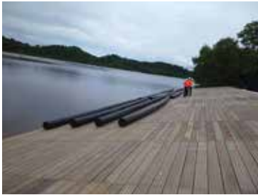
Floating pipes and metal structure
