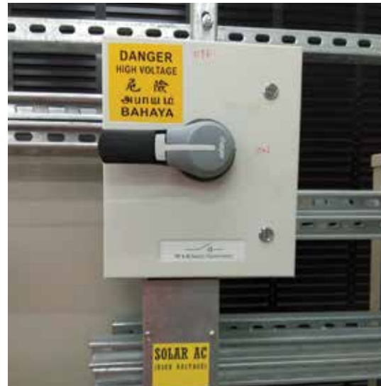
FIGURE 8.10 AC isolator
