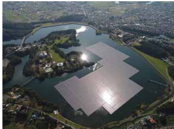
FIGURE 6.1 Glare on Yamakura dam in Japan
