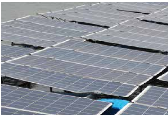
FIGURE 9.8 Replacement of a damaged solar module
