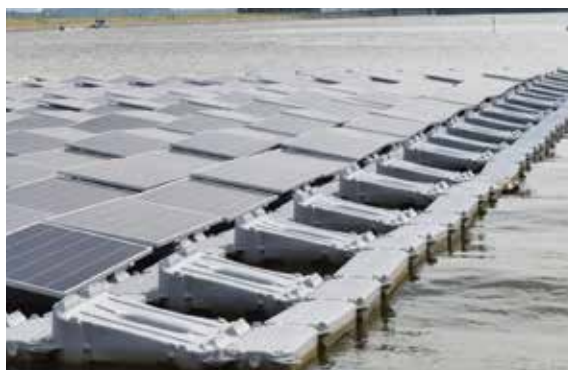
FIGURE 9.23 Varying tilt angle induced due to wind and waves
