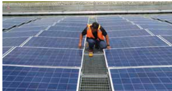
FIGURE 8.5 Solar professional performing continuity tests
