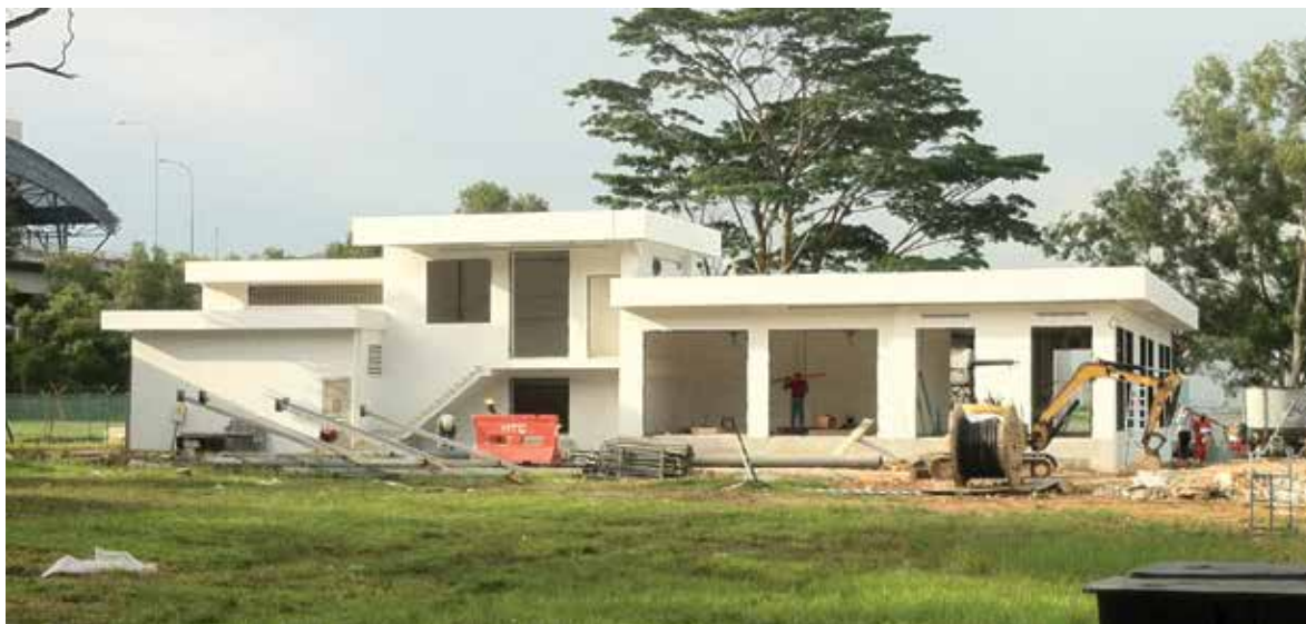
FIGURE 7.13 A substation under construction
