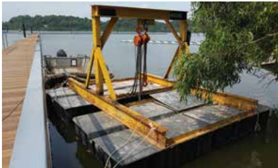
FIGURE 7.9 Barge used to lower concrete sinkers
