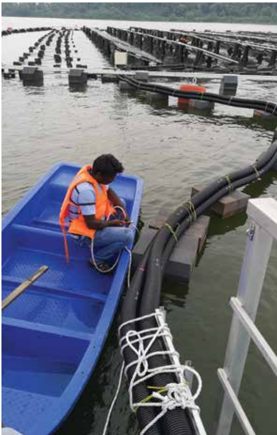
FIGURE 9.17 Maintenance on cables returning to shore
