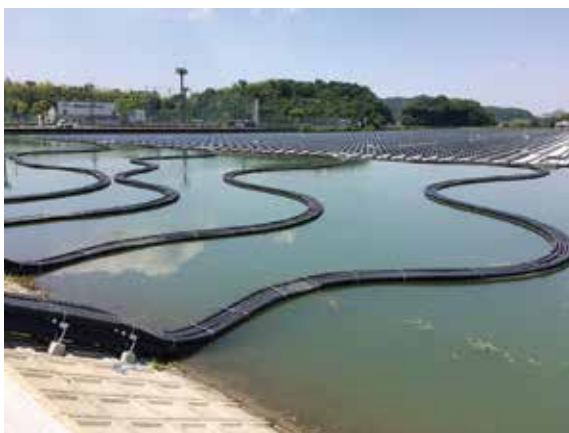
FIGURE 4.12 Cables routed to land from floating islands in MWp-scale FPV plants in Hyogo Prefecture, Japan (left), and in Anhui Province, China (right)
