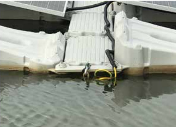
FIGURE 8.4 Grounding to reservoir bed
