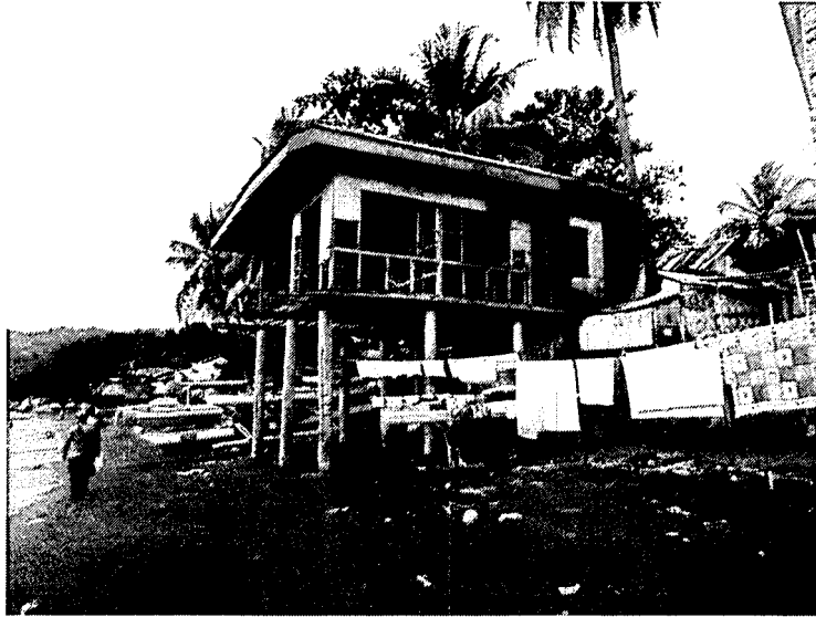
Fig. 35 Abandoned stilt house in Misamis Oriental. Elevated houses offer protection from inundation in the area.
