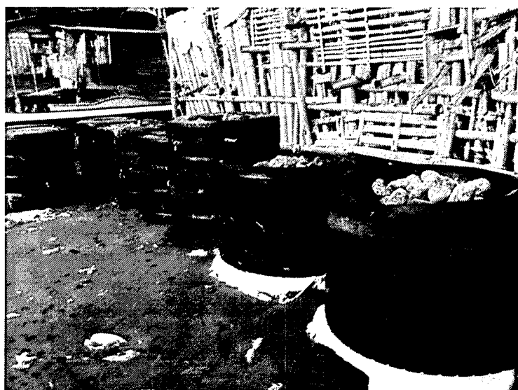
Fig. 34 Layers of rubber tires placed filled with rocks were seen in front of the houses in coastal areas of Misamis Oriental.
