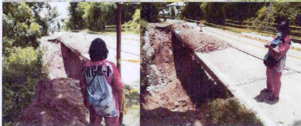
Figure 6 Scoured road sections along Barangay Mababayag, GPS Coordinates: 17°10'31.1" N, 120°30'37.5" E
