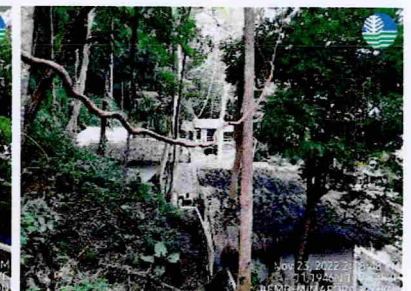
Villas that are under construction in the beachfront area
